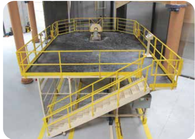
Operator Work Platforms
